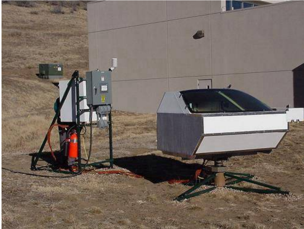
Figure 21. Mockup of passenger compartment for testing heat-pipe IP cooling
